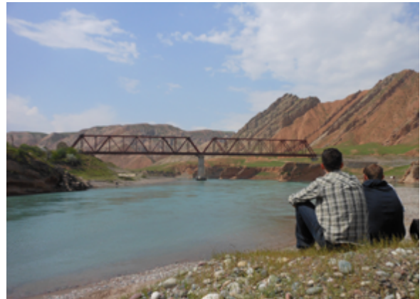
Train bridge over Vakhsh River Flickr / Christian
