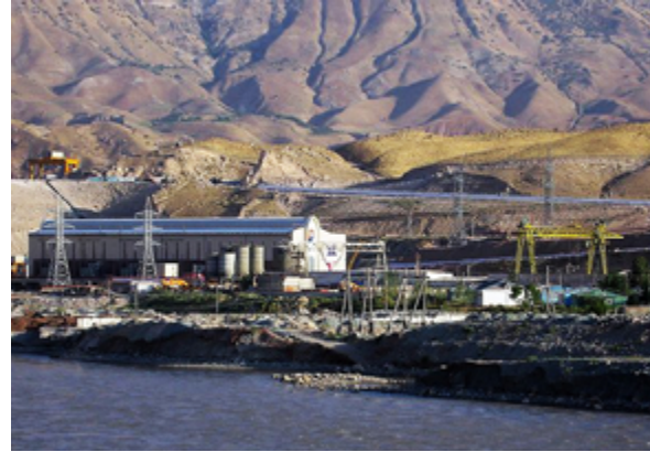
Sangtuda 1 hydroelectric power plant Wikimedia / Russian Presidential Press and Information Office
