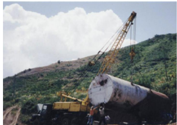
Constructing the fuel farm Wikimedia / Brian Harrington Spier
