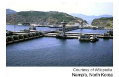
One of the largest projects in North Korean history was the construction of the West Sea Barrage ("the longest dam in the world") just west of Nampo, which separates the saltwater Yellow Sea from the freshwater Taedong River. Ships traveling to and from Nampo pass through a lock system. A primary goal of the project was to expand the
